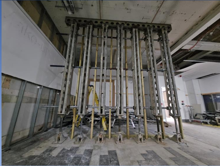
Installation of back-propping
