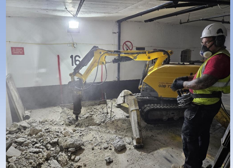
Basement Investigative Works
