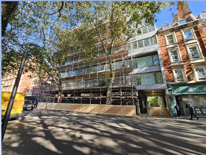
Scaffolding Erection on Gray's Inn Road
