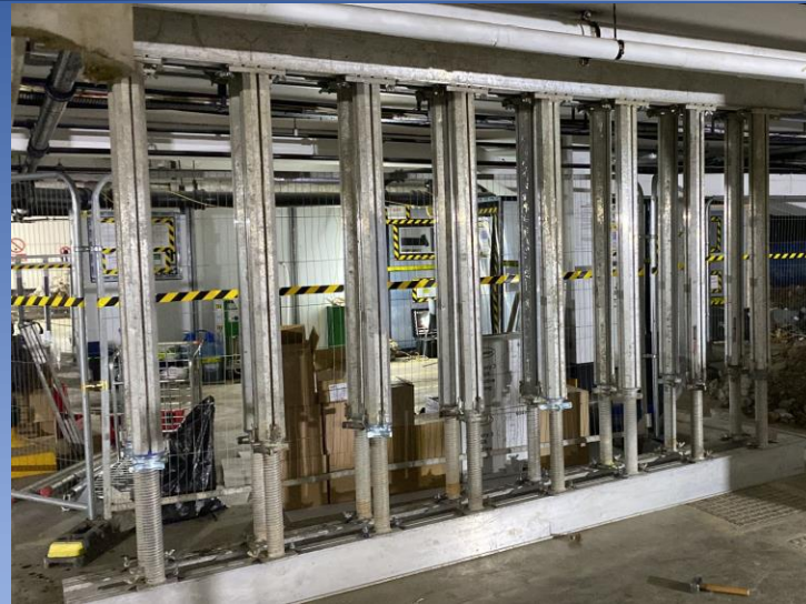
Installation of back-propping
