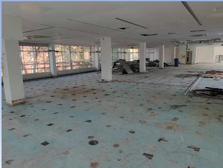
Typical soft-stripped floor
