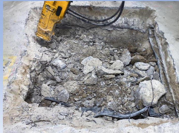
Basement Investigative Works
