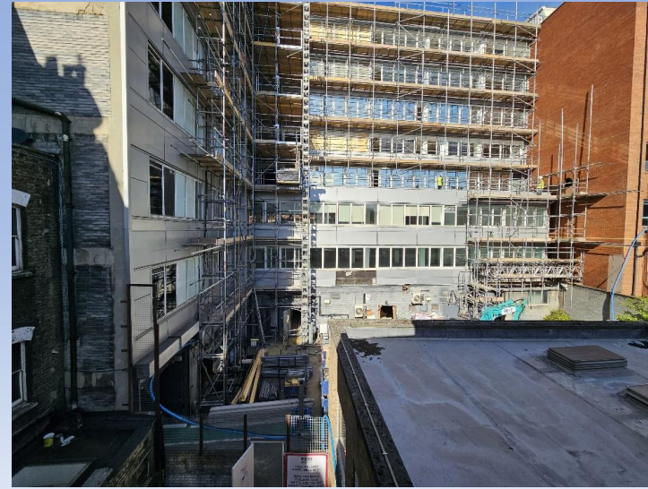
Scaffolding Erection to rear elevations
