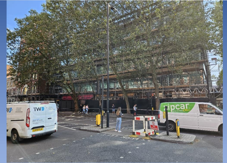
Scaffolding Erection on Clerkenwell Road
