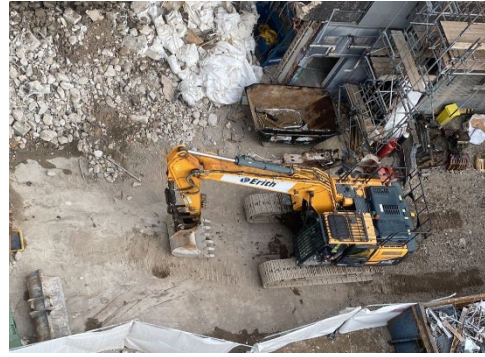
100 Gray's Inn Road courtyard logistics area.
