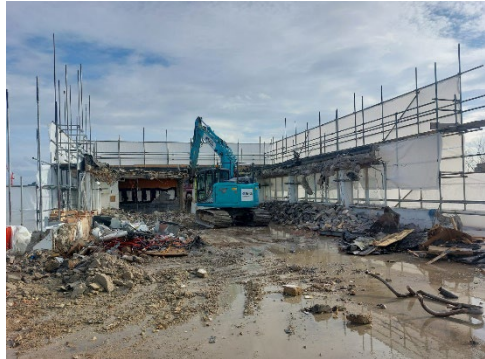
100 Gray's Inn Road: demolition of roof structure nearing completion.
