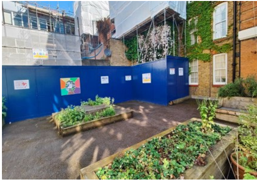
Hoarding erection within the quiet gardens
